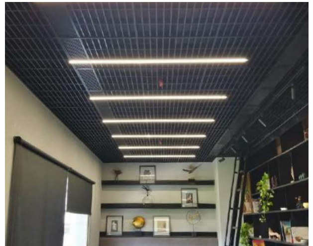
Reflected Ceiling Plan for METALIUM 150*150 Cell - T Grid Ceiling Systems
